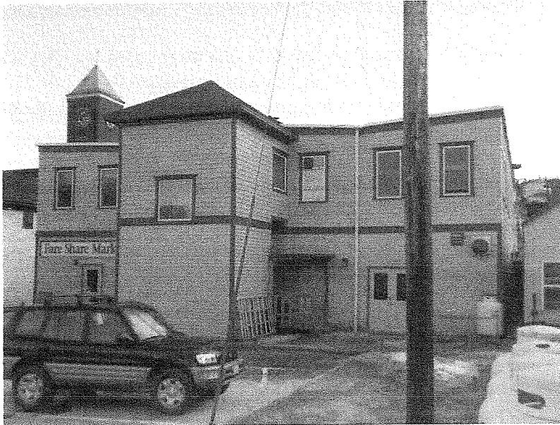
Figure 2: East Side of Fare Share Co-op Building
