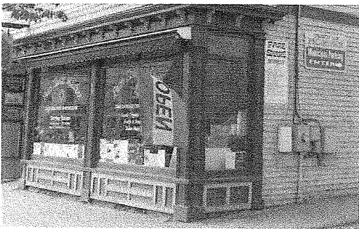
Figure 4: Single Pane Store Front Windows of Co-op
