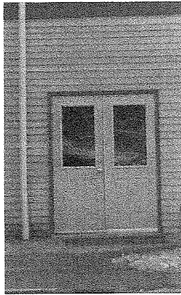
Figure 6: Co-op Loading Doors East Side of building
